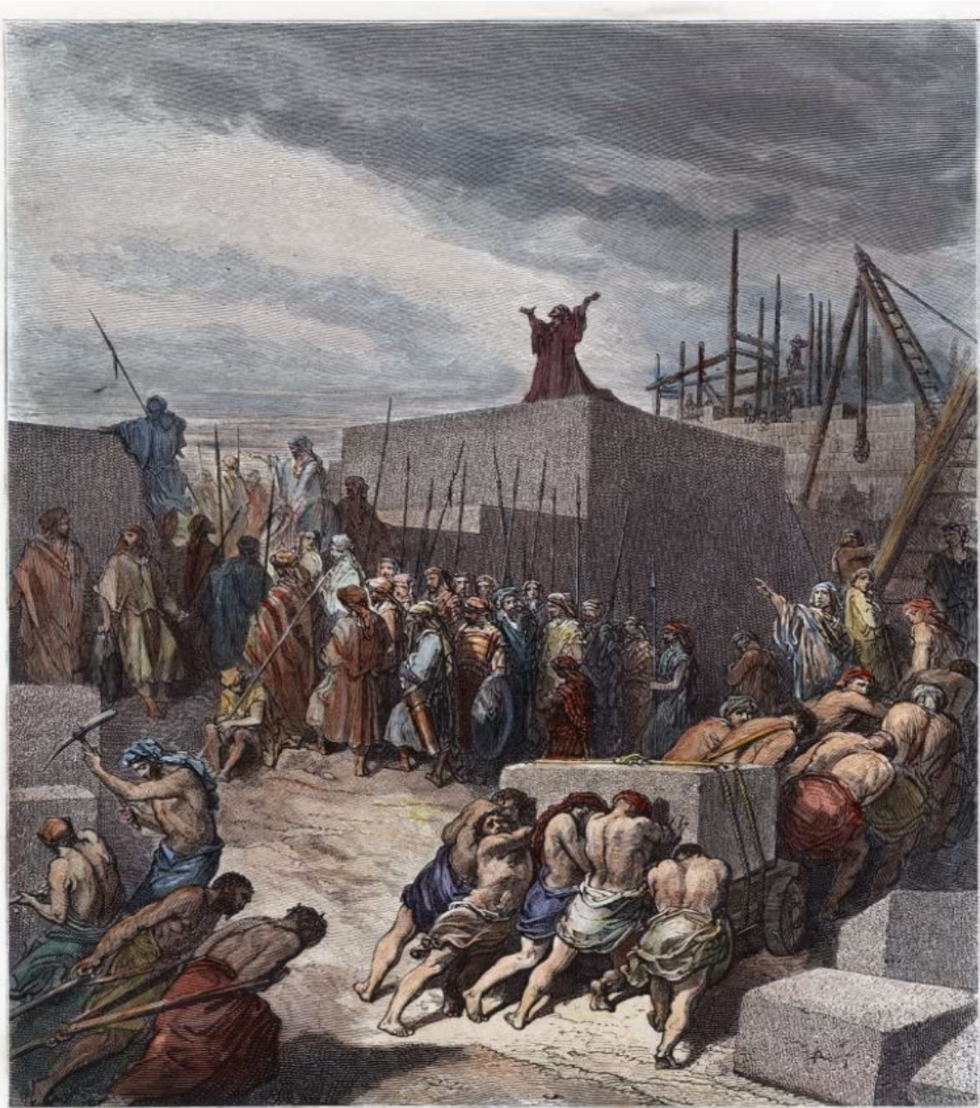
THE REBUILDING OF THE TEMPLE
